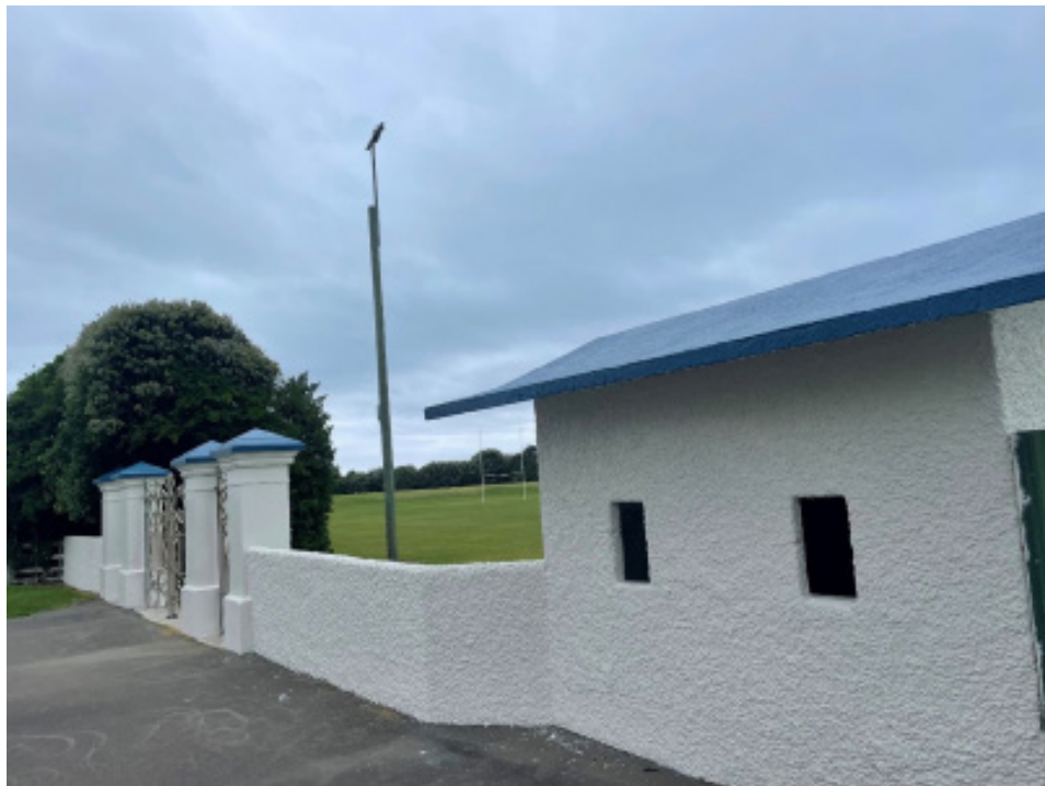
Above: Exterior of old Ticket Booth and Memorial gates, painted in Resene 'Half Tea', with 'Billabong' roof and tops of gate posts.
